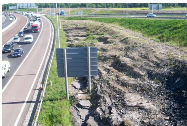
Close up of the road cut to the west of the access road, showing how benches have been created to reflect naturally occurring rock formations.
