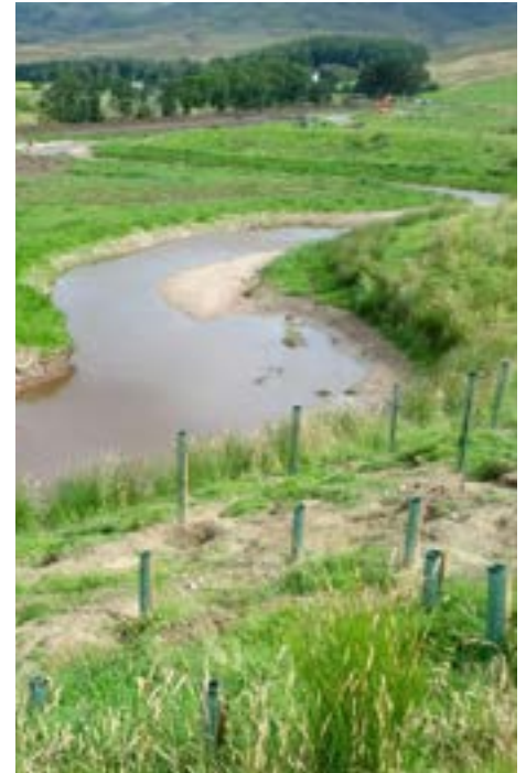
Restored meander at Rottal Burn, Glen Clova; creating a more natural flow benefiting habitats and wildlife. © EnviroCentre.
