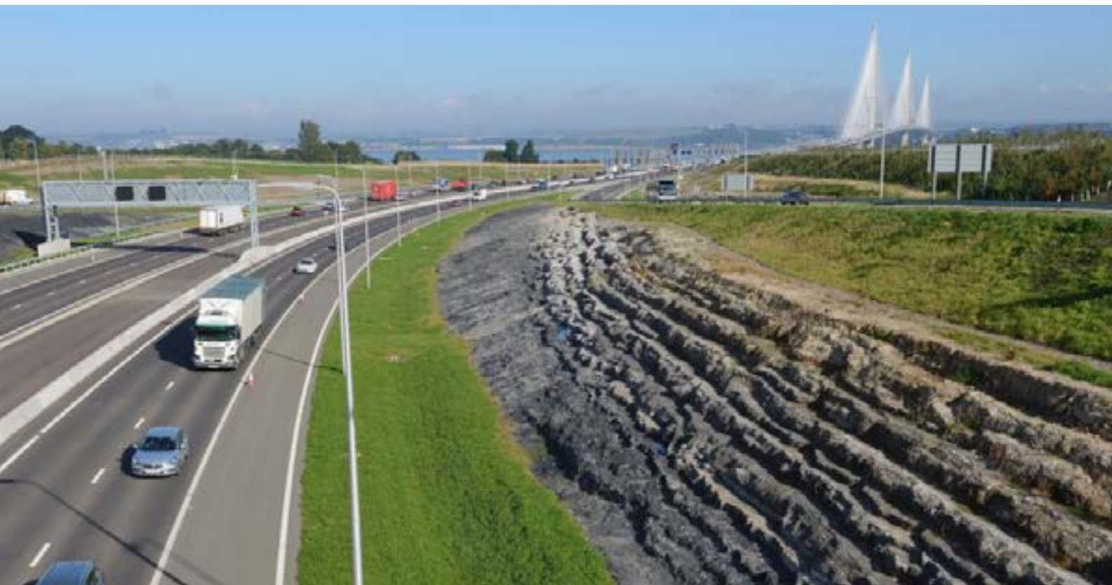
A new rock cutting on the southern approach to the Queensferry Crossing exposes a superb section through Carboniferous sedimentary rocks, including sandstone and mudstone. © Lorne Gill/SNH.
